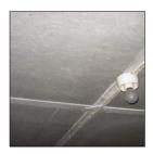
If the plates have paper on both sides and are made in a white gypsum material, it is gypsum which does not contain asbestos.
