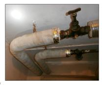
Asbestos material was often used in the period of 1955 to 1980, on pipe bends, pipe ends and pipe branches.
