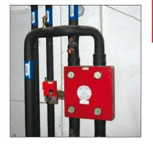
Cellular rubbers containing brominated flame retardants was used as insulation prior to 2003.
