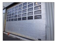
If the garage door is produced prior to 2003, the insulation foam is most likely very damaging for the ozone layer. The port/door needs to be delivered as hazardous waste.
