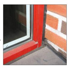
Sealant produced between 1960 and 1978 usually contains PCB. From 1970 to 1990, chlorinated paraffins was used. Both substances are harmful to the environment.
