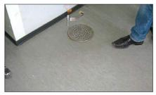
of tiles are often used in staircases, hallways and in kitchens. Vinyl is the same as PVC. Also pay attention to the glue used to attach the vinyl. If the glue is black and used between 1950 and 1970, it can contain asbestos.
