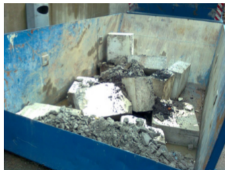
Malt betong Foto: Norconsult AS
